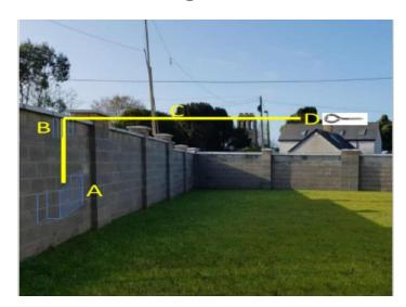
Feed **C** up through **A** across to **B** and secure at **D**.
